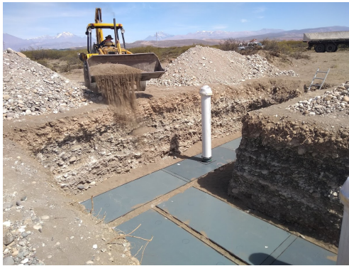
Figure 1: Left: Modules are buried, the tubes give access to the electronics dome from the surface for maintenance and repair. Right: Electronics dome of a UMD module before is closed, it can be observed how the optical fibers carry the light to the cookie where the SiPM array is afterward placed.
