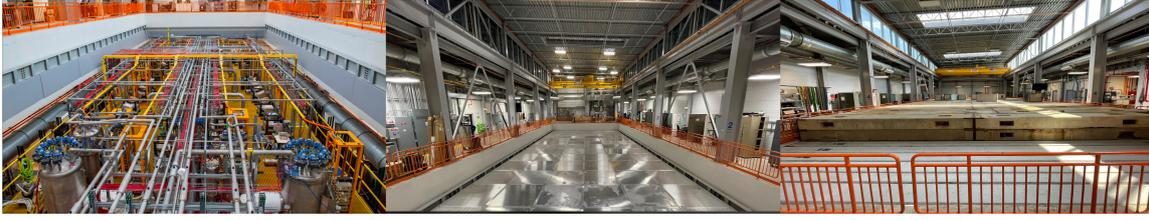
**Figure 1:** Assembly activities in the ICARUS detector: left shows TPC, PMT and part of the cryogenic subsystems installed, middle picture the fully completed CRT and finally the blocks of concrete overburden being put into place on the right.
