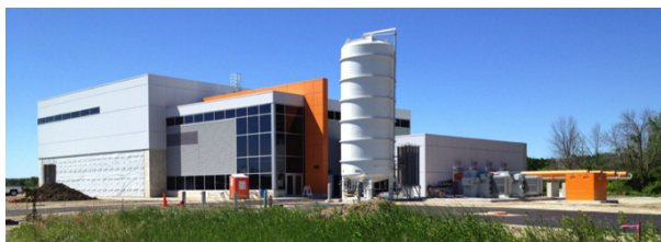
Figure 3: The new MC-1 building at Fermilab, where the muon g-2 storage ring is being reassembled in the larger part to the left. The part to the right houses the counting room, electronics, etc, with cryogenics services further right. (Image credit: Fermilab.)
