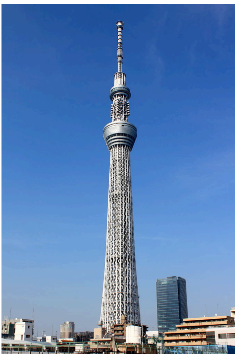
Figure 2. The Tokyo Sky Tree tower (634m), which opened in May 2012.
