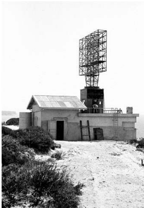
Fig. 1. The shore defence radar of the CSIR Division of Radiophysics from WWII, used on 26 January 1946 for the first interferometry in radio astronomy by Payne-Scott. The small angular size of the solar bursts was determined. From the CSIRO Radio Astronomy Image Archive.
