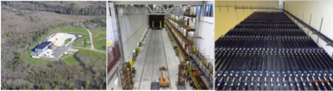
Figure 5: Aerial view of the FD (left), the 2 nd block transported to the far end of the FD hall (center), and a top view of the first two blocks showing a total of 64 layers (right).
