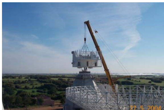
Figure 7: Lifting the fork of the 40 meter IGN radiotelescope.
