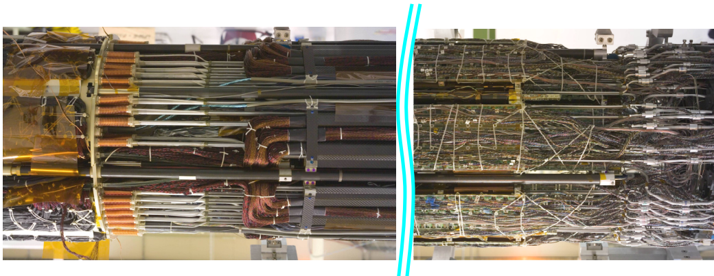
Figure 1: Composite image of service connections for one of the ATLAS pixel detector.
